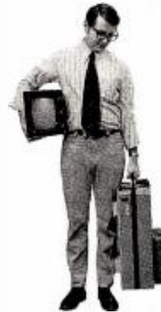
Easy-to-carry TK-630 color camera with plug-in detachable viewfinder becomes a portable at moment's notice.
